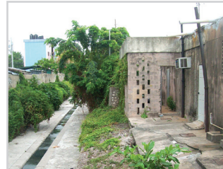
Photo 3: Rear of the station without security fencing as seen on June 29, 2012.
