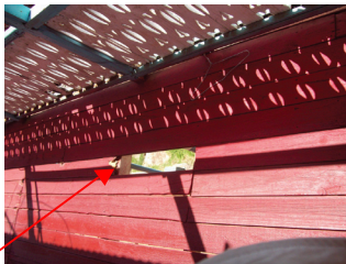
Photos 5 & 6: Missing floor boards at the Mocho Station as seen on March 19, 2014.
