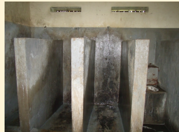
Photo 8: Bathrooms at Hunts Bay Station lock-up.
