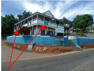
Photo 1 & 2 Missing rails at the Mocho Station as seen in 2012 and 2014.
