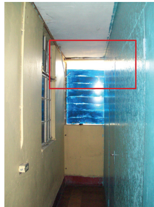
Photos 3, 4 & 5: Missing windows in Station building as seen on August 20, 2013.
