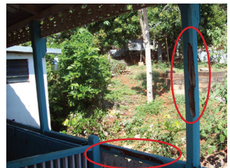
Photos 7 & 8: Rotting rails at the Mocho Station as seen on March 19, 2014.
