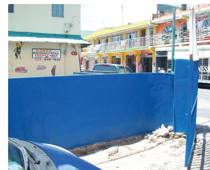
Photo 10: Low perimeter wall at the Rollington Town Station on September 19, 2013.
