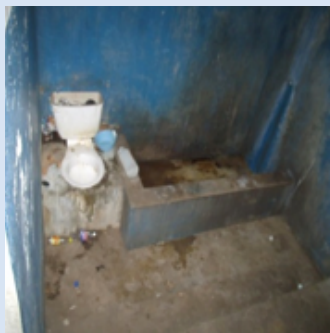
Photo 5: A view of bathroom at Castleton Station.
