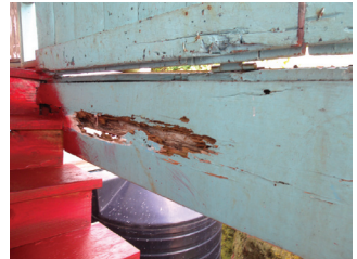
Photos 3 & 4: Rotting wood along staircase at the Mocho Station as seen in 2012 and 2014.
