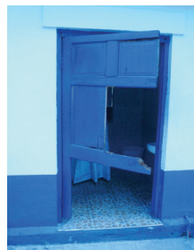
Photos 13 & 14: Kitchen and Bathroom doors in need of replacement at the Frankfield Station as seen on March 20, 2014.
