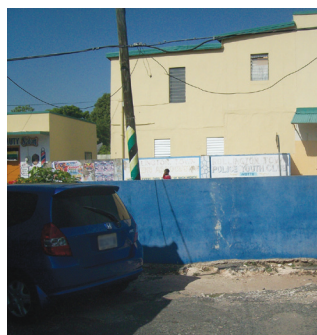
Photo 9: Low perimeter wall at the Rollington Town Station in September 26, 2012.
