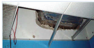
Photos 5 & 6: Missing ceiling tiles, exposed electrical wire and water marks on ceiling at the Grants Pen Station on November 7, 2013.
