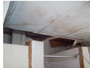
Photo 3: Torn away section of ceiling.
