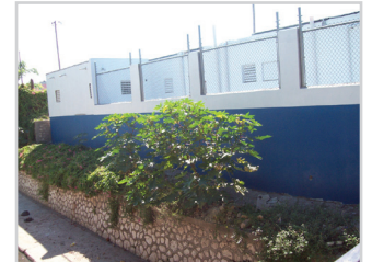
Photo 4: New security fencing at the rear of station as seen on March 13, 2014.
