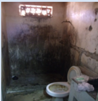
Photo 4: A view of the bathroom at Barrett Town Station.
