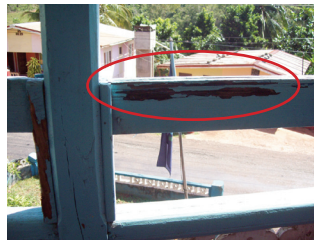
Photos 7 & 8: Rotting rails at the Mocho Station as seen on March 19, 2014.
