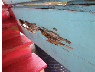
Photos 3 & 4: Rotting wood along staircase at the Mocho Station as seen in 2012 and 2014.
