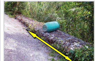
Photo 2: Absence of perimeter fencing at Gordon Town Station as presented November 12, 2013.
