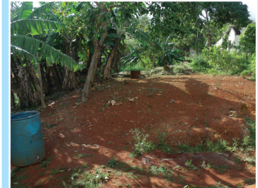
Photo 4: Absence of perimeter fencing at the Newport Station.
