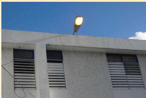
Photo 3: Security light on during the day at the Golden Grove Station on November 27, 2014.
