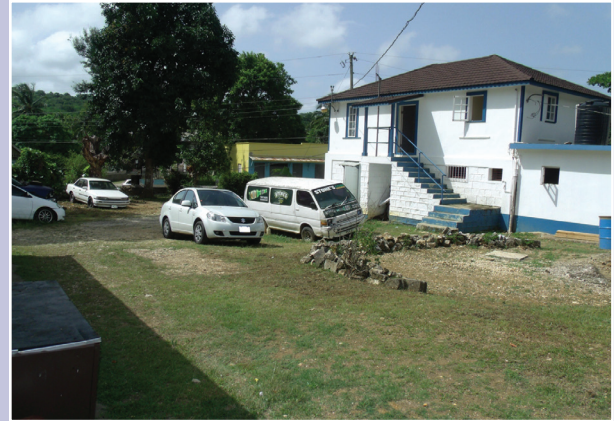
Photo 3: Absence of perimeter fencing at the Adelphi Station seen on July 2, 2014.
