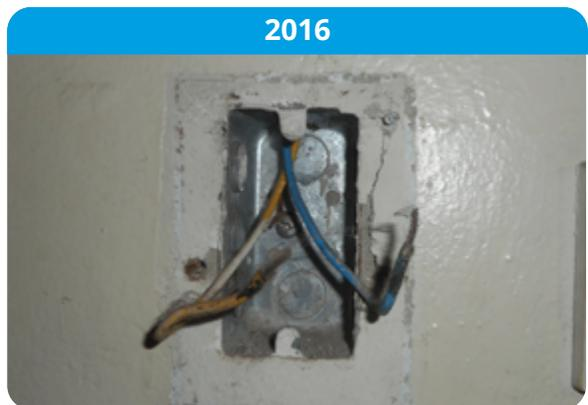
Unsecured electrical wires at the Gold Street Station as seen in 2013 and 2016
