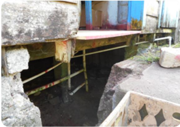
**Rotting floor and leaking ceiling at the Belfield Station**
