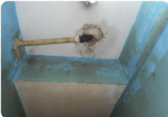
Leaking pipe at the Annotto Bay Station with bucket to catch waste water
